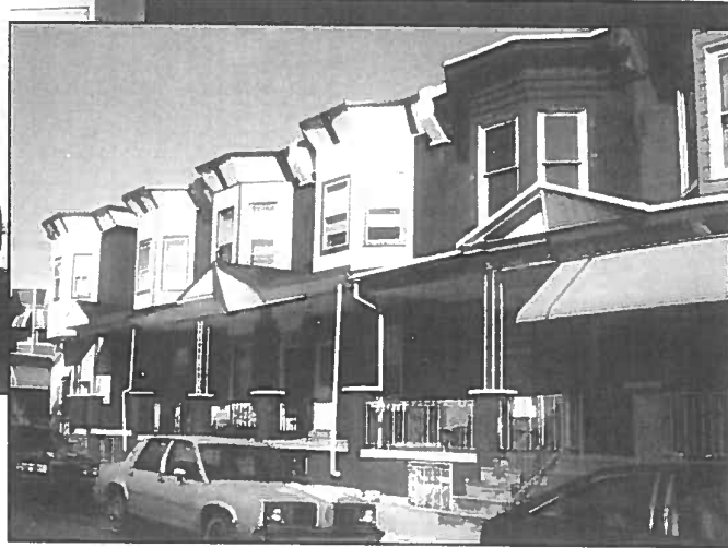
Rehabilitated property, exterior
