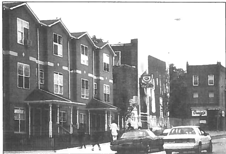
New construction, Diamond Street Corridor area
