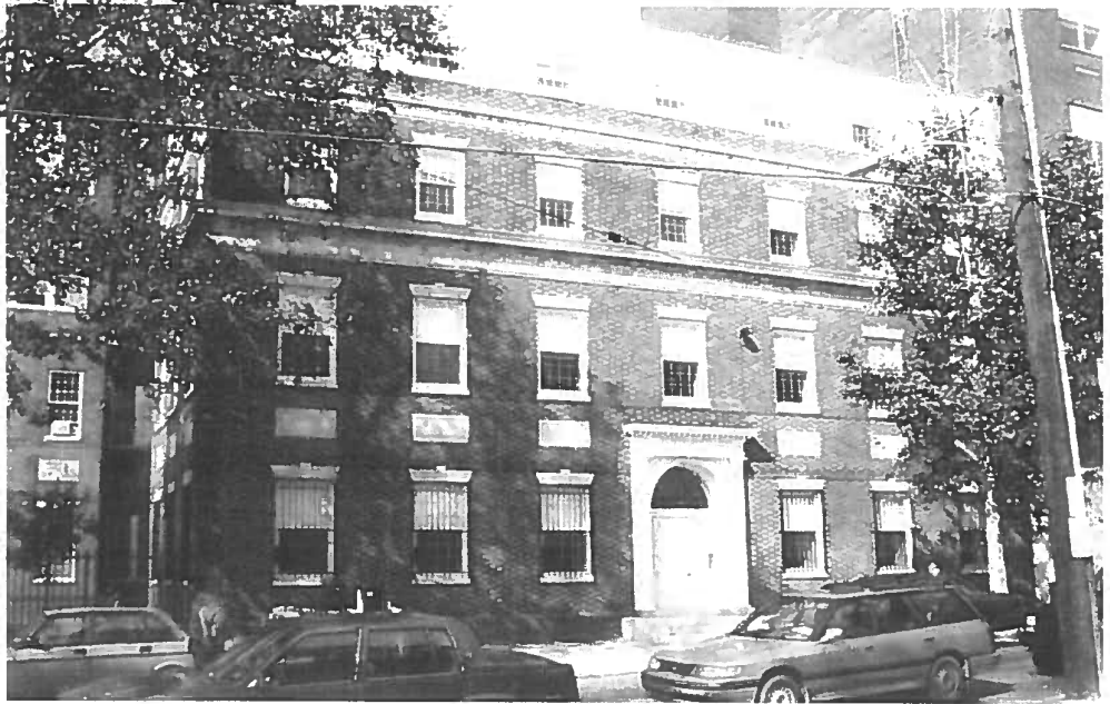
Lehigh Park Center, Lawrence and Huntingdon Streets
