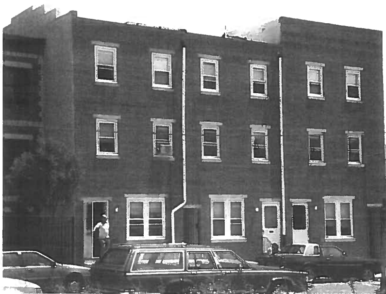
PHA scattered-site houses rehabilitated by PHDC.
