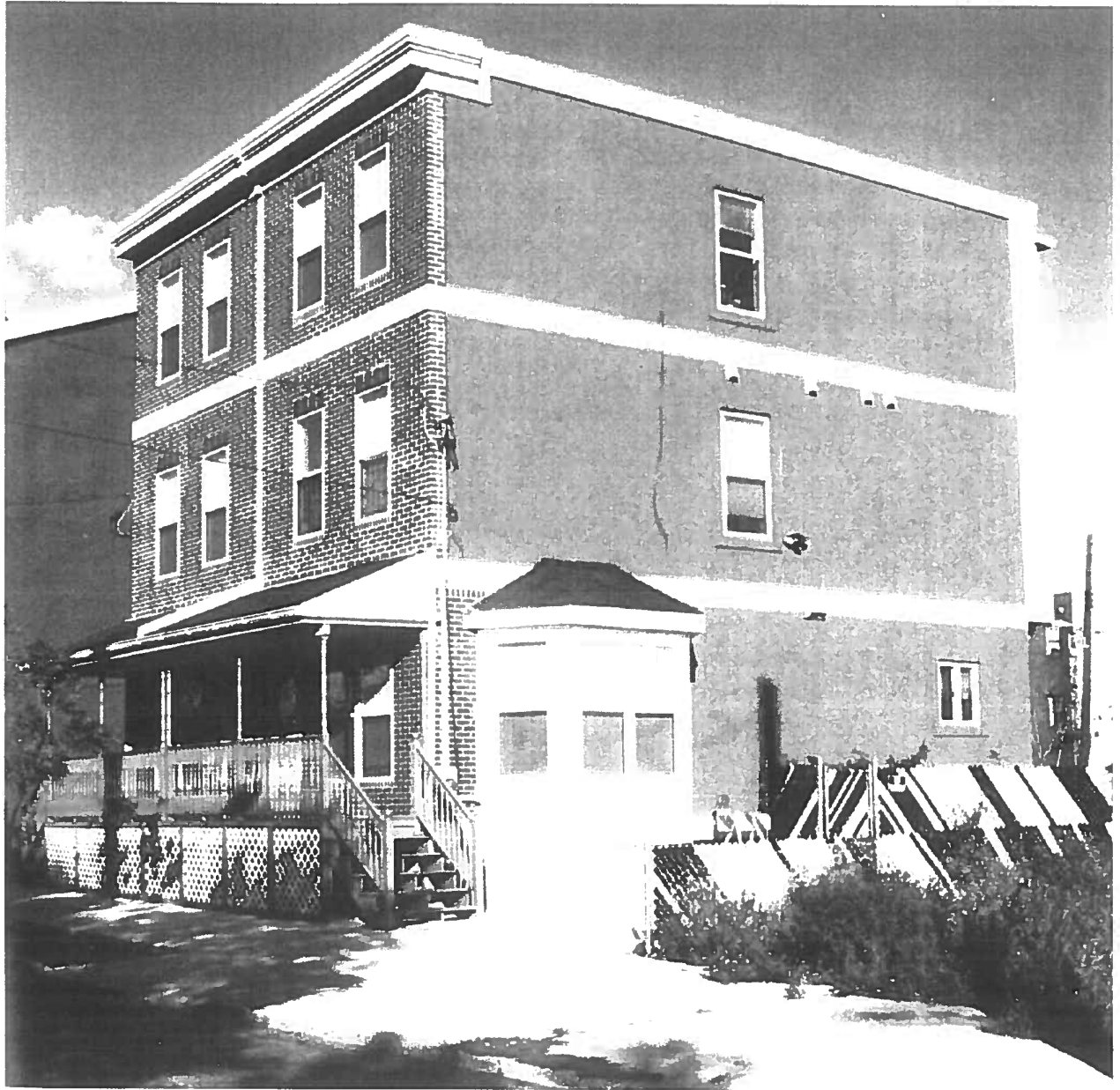
Ludlow Phase I townhouses
