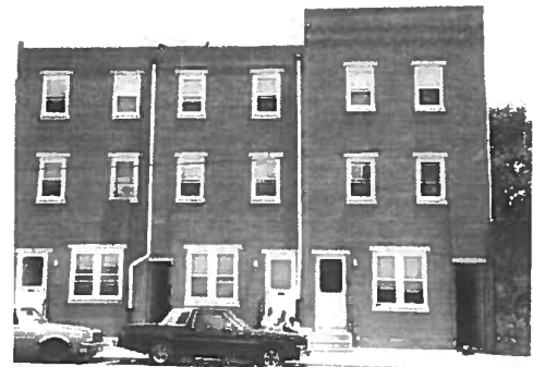
Rehabilitated public housing adjacent to One APM Plaza
